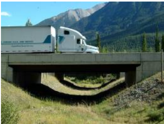
Figure 5.26: Wildlife underpasses (National Cooperative Highway Research Program (NCHRP))
