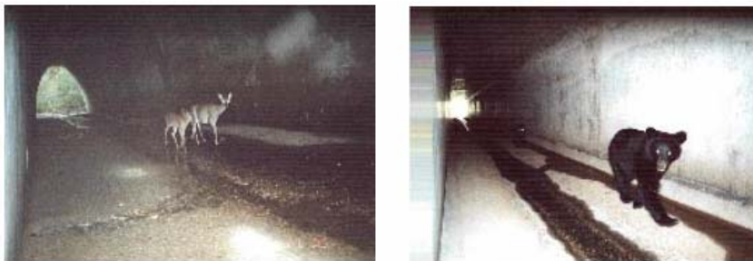
Figure 3.2: Large Mammals passing through box culverts
