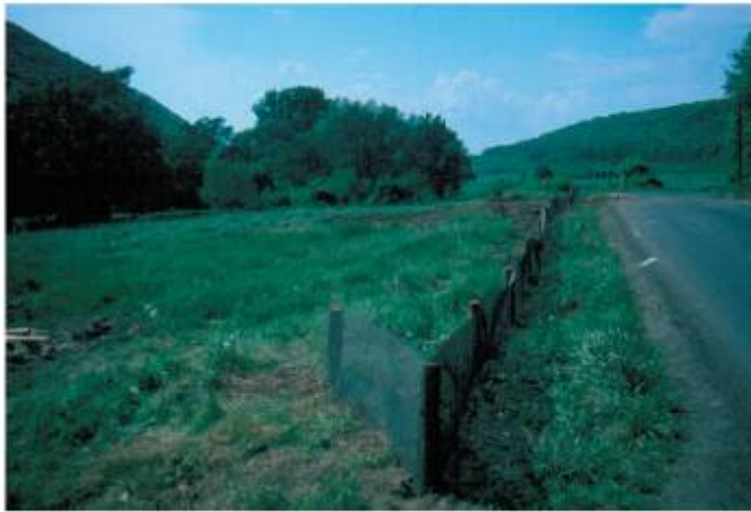
Figure 5.6: Fence for small animals and amphibians with turned-back end to prevent animals from approaching the road (Puky, 2003)
