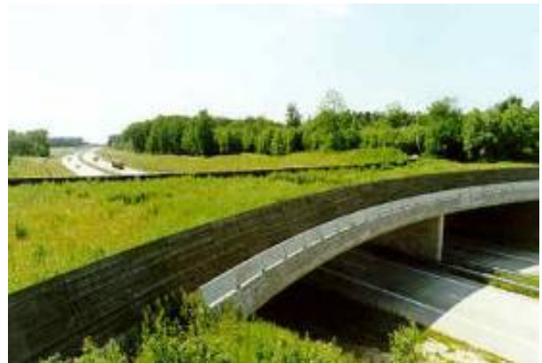
Figure 5.31: Wildlife overpass, or "green bridge" (NCHR)
