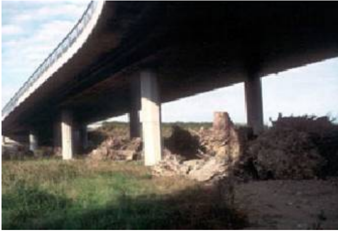
Figure 5.23: Underpass to accommodate large and medium mammals, with stumps and vegetative cover for small animals (FHWA/US DOT, 2002)
