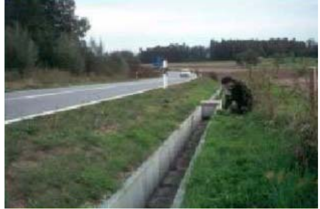
Figure 5.5: Concrete trench and drop inlet with one-way pipe for amphibian crossing (FHWA/US DOT, 2002)
