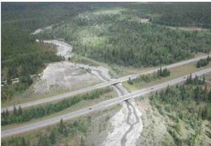
Figure 5.24: Creek underpass in Banff National Park, Canada (Clevenger, 2004) http://www.pc.gc.ca/pn-np/ab/banff/docs/routes/chap1/sec1/routes1b_e.asp
