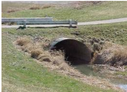
Figure 3.10: Culvert with standing
