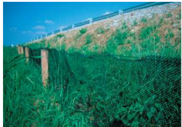
Figure 5.3: Fine plastic mesh fence for small animals and amphibians (Puky, 2003)
