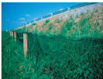
Figure 3.4: Fine mesh fence for small animals
