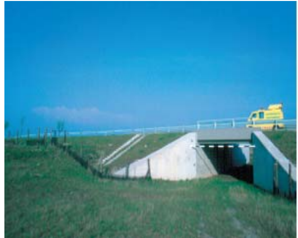
Figure 5.16: Box culvert underpass and fencing for multiple species (Puky, 2003)
